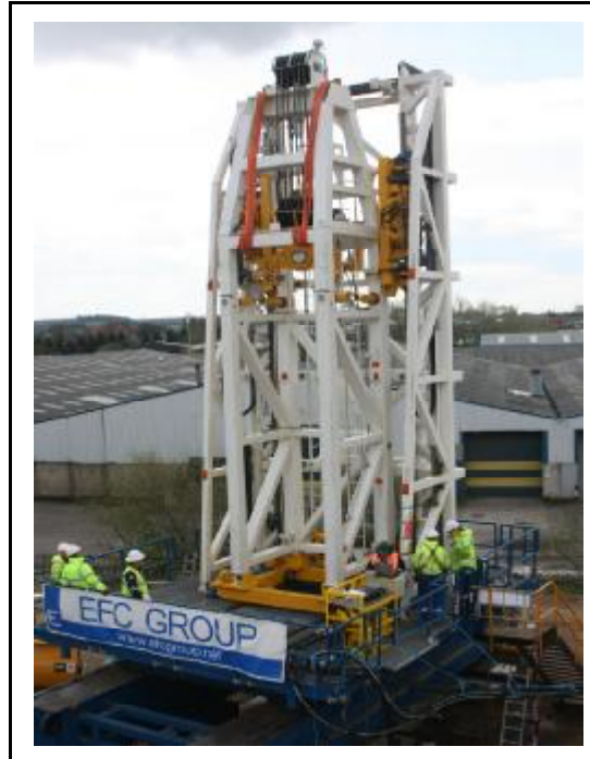
Crown & 1 st Mast Connected (Locking Bolts in place)
