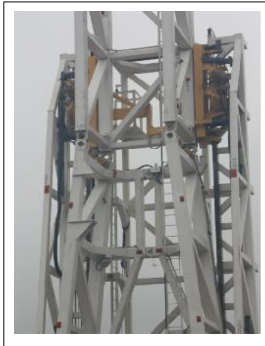
Crown, Masts 1, 2, 3 & 4 being Lowered onto Base Mast
