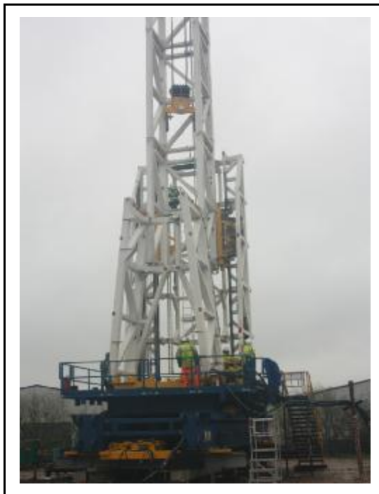
Crown, Masts 1, 2, 3 & 4 being Lifted, Base Mast on Cross Travel Carriage
